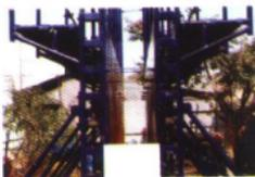
Consists of wallform panels made out of 12 gauge Sheet and M.S. Angle / Flat Frame, channel / Heavy Duty Soldiers, Tubular/Channel waters & accessories. Panels supplied in 1.25m & Soldiers in 2.5m heights. For curved walls, flexible panels are used, and heavy duty soldiers to be used in place of channel soldiers for single side shuttering.
